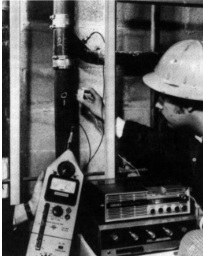
FIG. 7 — Testing a Hubless System During Constructon of the Massachusetts House
