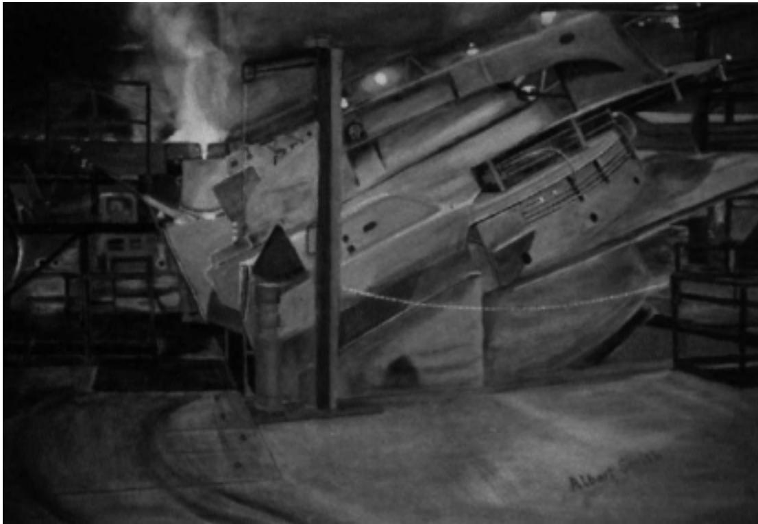
FIG. 4 — Mixing Ladle Located in Front of a Cupola
