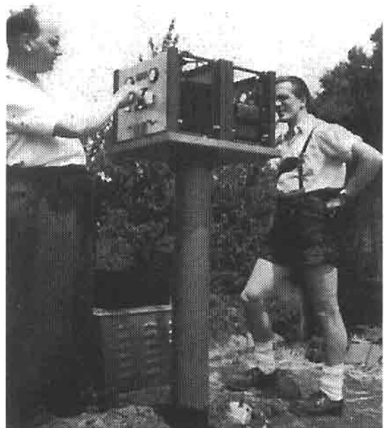
Fig. 1-14 Cathodic protection rectifier manufactured in France (1952) at Bogenheim in the Palatinate.
