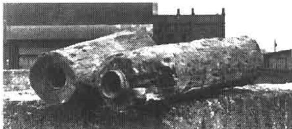
Fig. 1-3 Oak water pipe over 200 years old laid above ground in the Wadgassen Abbey (Saarland) with cast iron clamps (photo: Mannesmann Archives).
