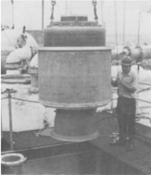
FIGURE 6 Ship-loading cryogenic pump (J.C. Carter Company, Inc.)
