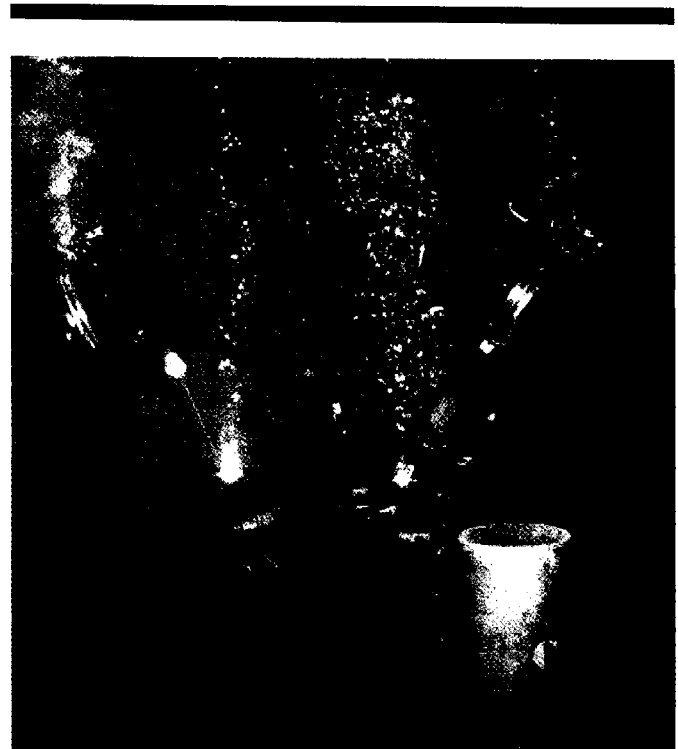
Figure 10.12—Welder/Dividers Repairing Offshore Structure Using Underwater Wet Welding
