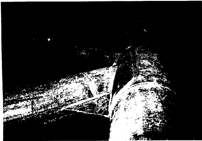
Figure 10.1B—After Underwater Wet Welded Repair, Offshore Structure K-Brace is Sound
