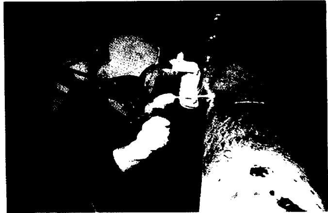
Figure 10.2—Welder/Diver Repairing Offshore Drilling and Production Platform at Depth of 320 ft (100 m)
